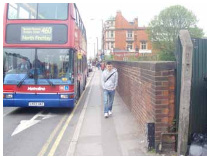
The bridge over the railway lines
